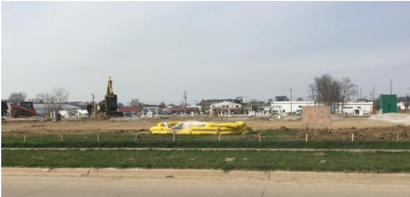
Access Center construction site 4/10/20
